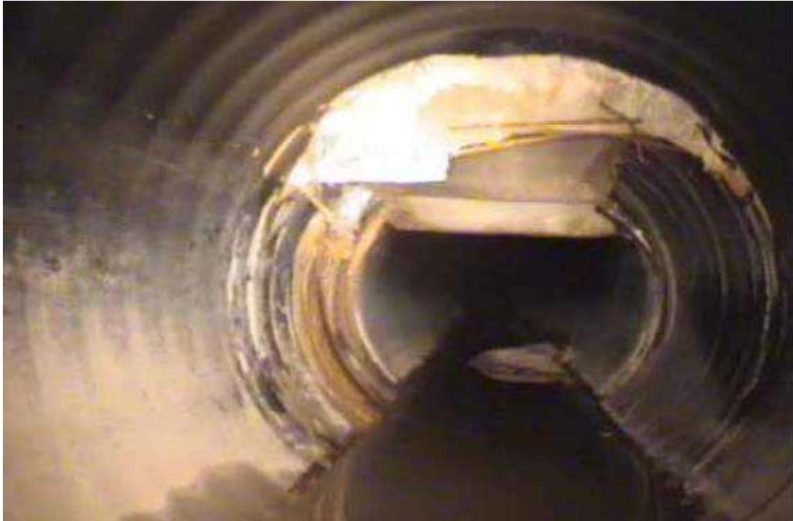
Figure 14. Joint displacement, cracking/fracture, and inverse curvature failures for pipeline in Houston, Site 8 [19]
