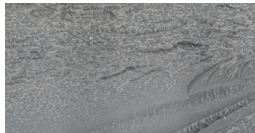
Figure 15: U-PVC structure after break
