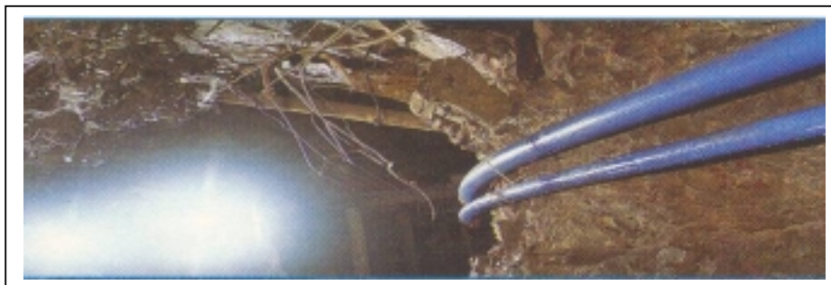
Figure 1. Chilled water pipe installation in a mine haulage way.
