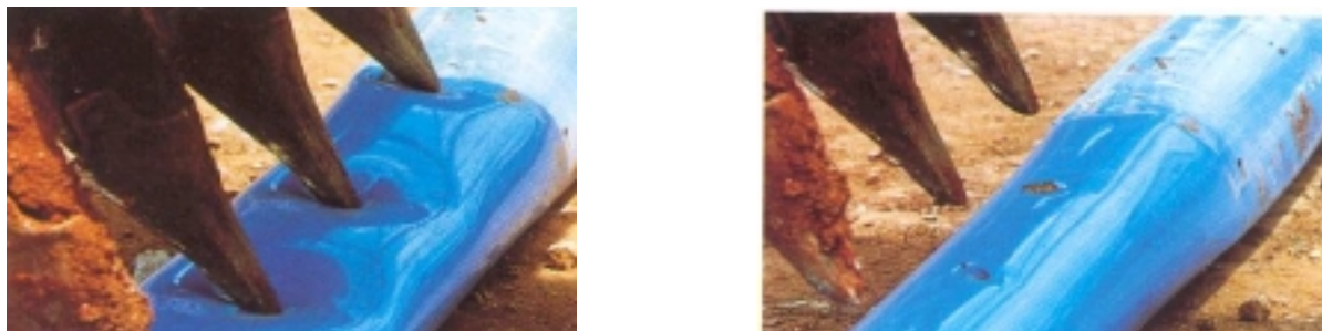
Figure 5. A construction site illustration of the toughness properties of PVC-O pipes.
