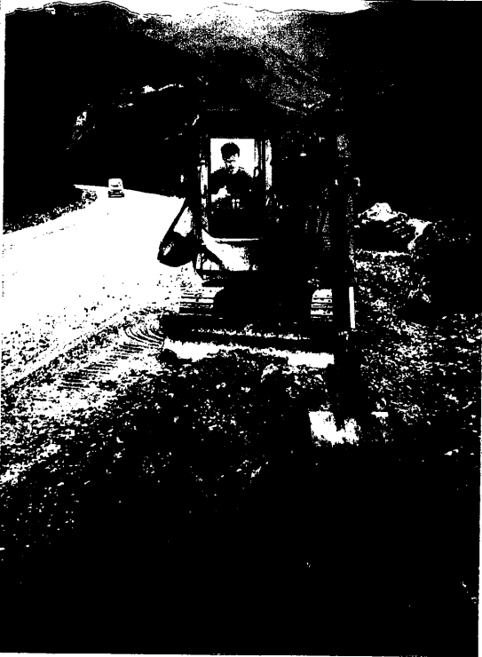
Digging in the French Alps, Courchevel. ▲
